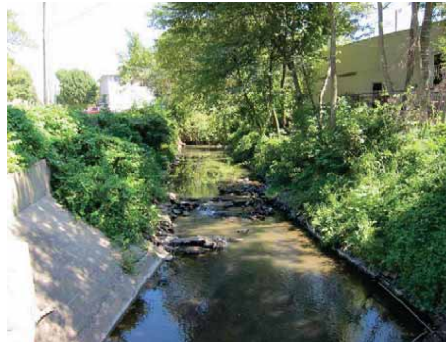
Creek Restoration to return Ralston Creek to an amenity for the area.
