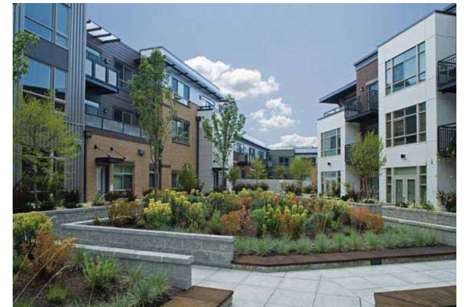
A senior housing development Merrill Gardens is located in Seattle near the University of Washington campus. The community consists of 123 independent retirement and assisted living apartments with a combination of studios, one bedroom and two bedroom apartments.
