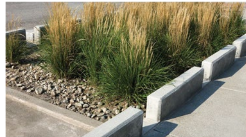
The bioretention planting areas will collect, cleanse, slow, and infiltrate storm water.
