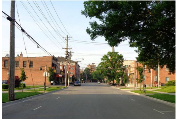
Existing conditions North Linn Street
