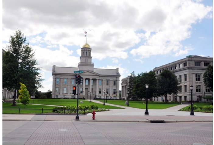
Existing conditions Iowa Avenue
