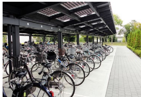
Bicycle shelter equipped with solar panels
