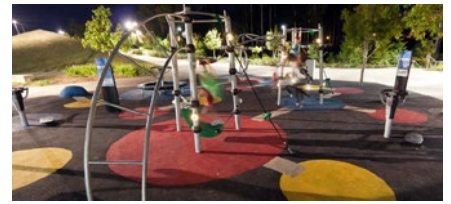
New Resilient rubber surfacing at existing play structure
