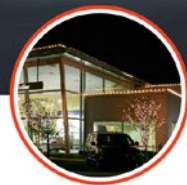
FIXED ARCHITECTURAL ACCENT LIGHTING
