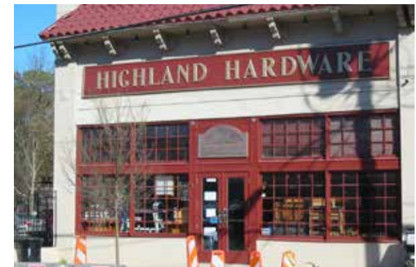
A correctly proportioned sign panel can work well within the defined sign band.
