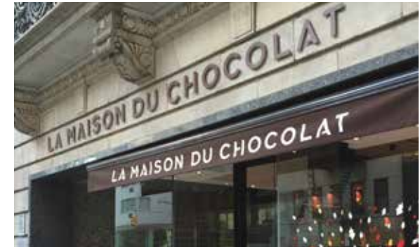
Individual letters that are proportional to building details can be an elegant fascia sign solution.
