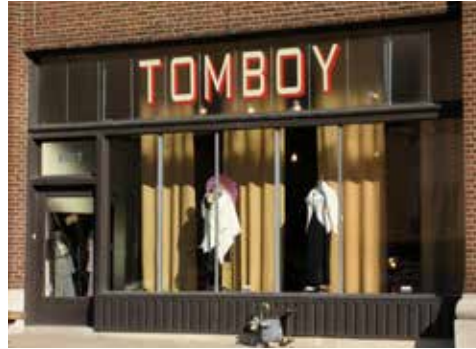
Window signage at the transom can be a good solution for providing store identification closer to pedestrian eye level.
