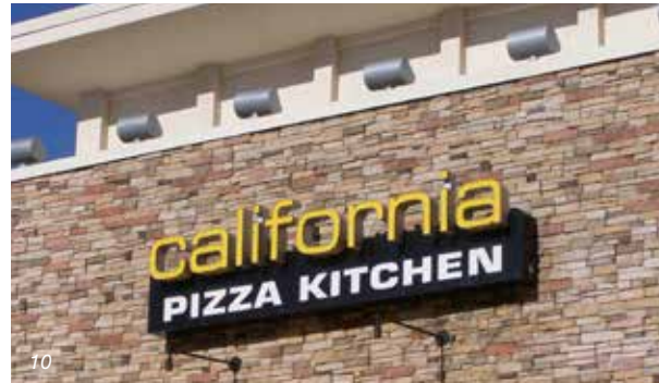
When no defined sign band exists, signage should be sized to work with the proportions of the building and other storefront elements.
