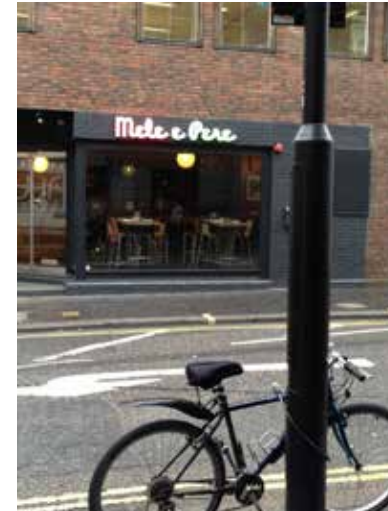
A window added to the secondary facade of a building uses paint to create a visually cohesive storefront.
