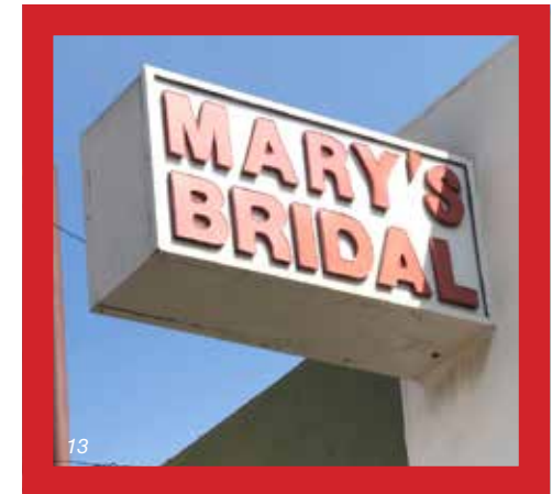
Internally illuminated, plastic-faced sign cabinets are not allowed. Signs should be mounted away from the building.
