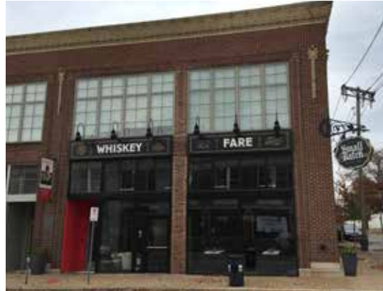
New retail in an old manufacturing building uses the proportions of the existing architecture to inform the renovated storefront design.
