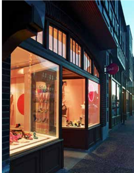
Transom windows not only allow light to flow in during the day, but help create a brighter, more dramatic storefront.
