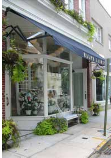
Placing signage on the valance of a retractable awning allows for visibility when the awning is closed.
