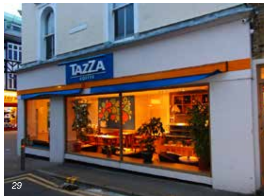
Retractable awnings can be pulled up in the evening to allow better views in and out of storefront windows.
