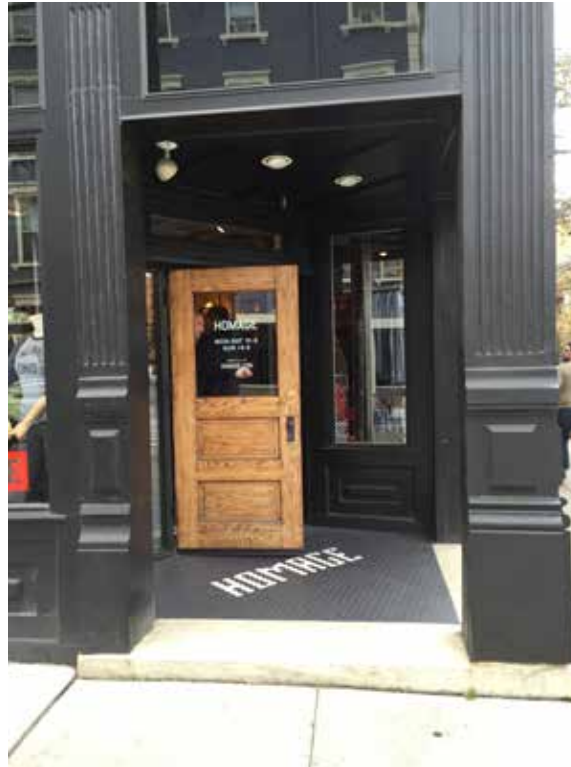
Doors should reflect the overall character of the building.
