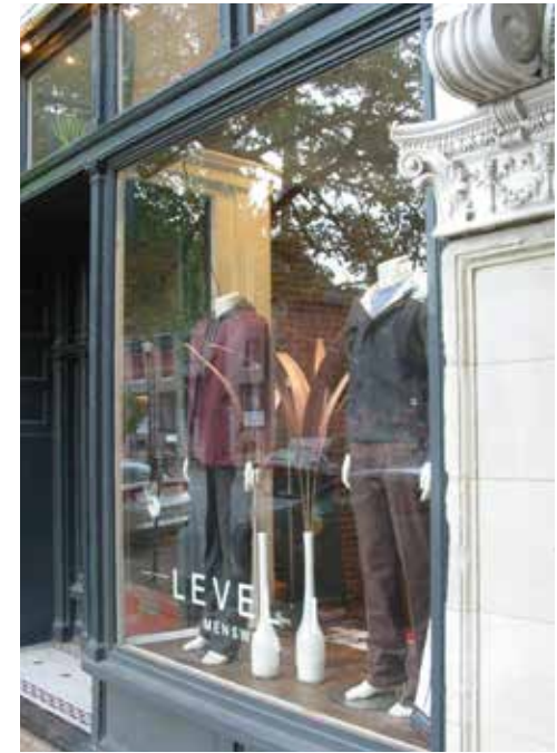
Knee walls provide a stage for merchandising.
