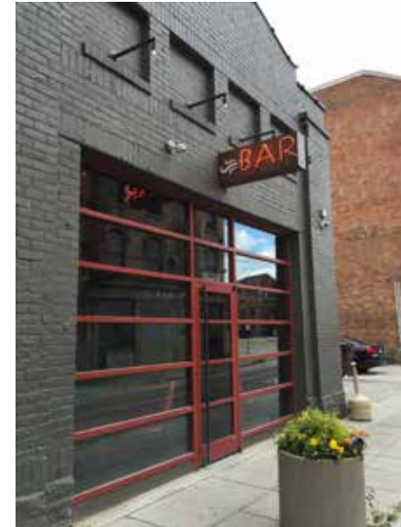
A creative storefront added to an old auto garage building is a play on garage door proportions.
