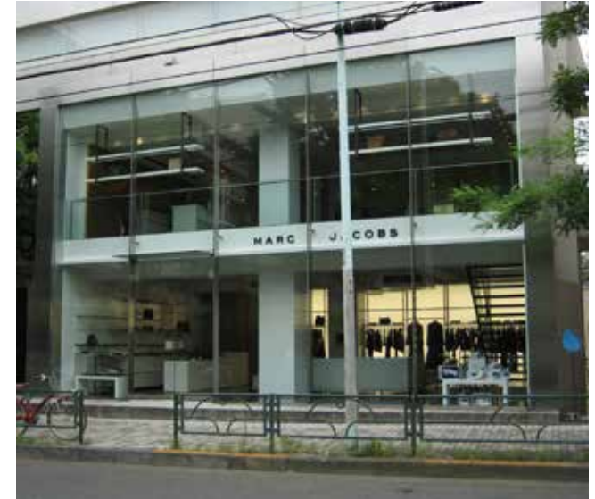
The interior spandrel panel behind this all-glass storefront provides a perfect sign band for the retailer.
