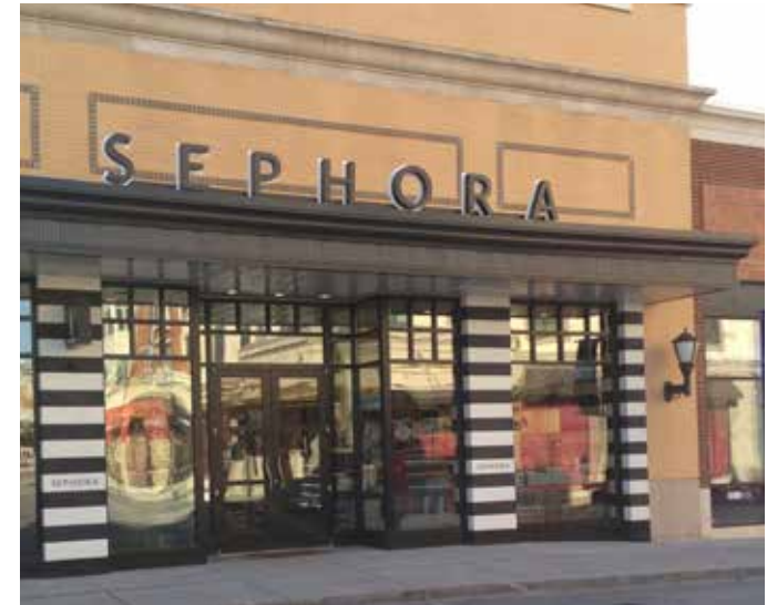
Canopies can serve to define a storefront and provide a location for signage.
