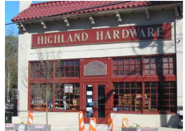
A correctly proportioned sign panel can work well within the defined sign band.
