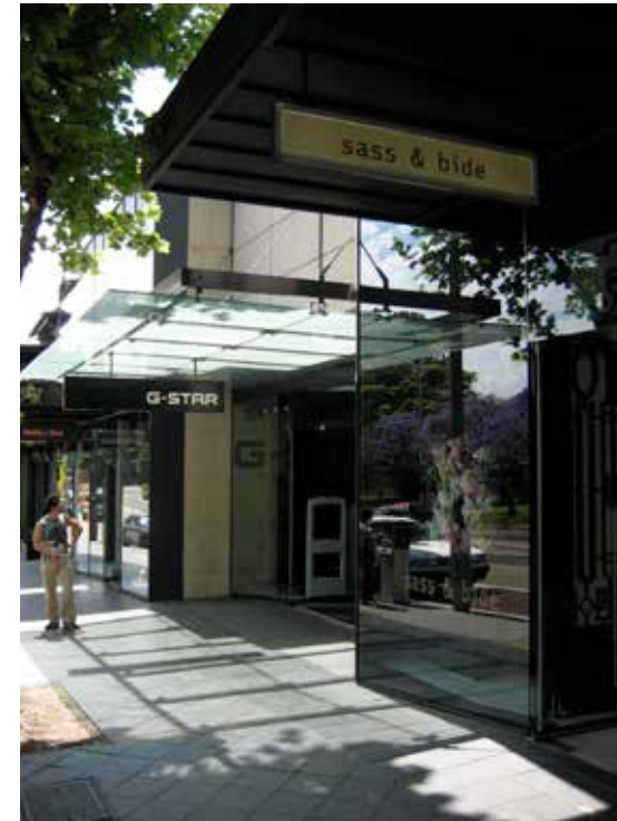
Canopy signs are a highly visible way to provide signage for clean modern storefronts. Canopies help to call attention to the entry doors.
